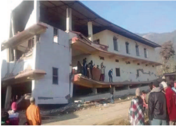
Fig. 4 Collapsed women market in Saikul
