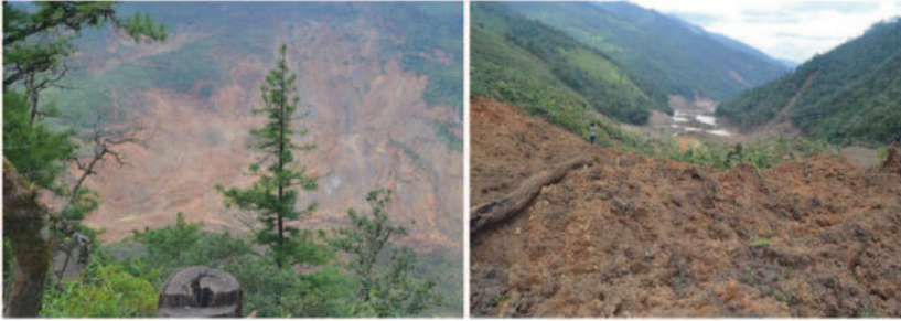
Fig. 3 Joumol village after the landslide (Photo: Michael Lunminthang)
